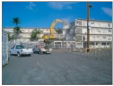
demolishing and downsizing more than 250 buildings (2 million square feet) existing on Johnston Island. Parsons also sorted, transported, placed, and backfilled over all demolition debris on the island and staged recyclable materials for off-island transport.
