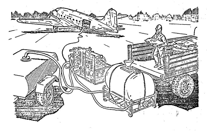
Figure 58. Mixing/Filling Operation with Wettable Powders
