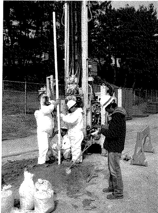
Photograph 9 – Monitoring well installation at Building 326 Investigation Area
