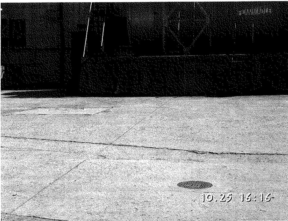
Photograph 4 – Newly installed monitoring well near AST adjacent to Building 326
