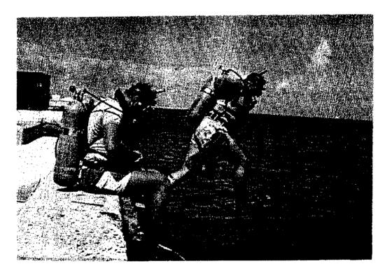
PLATE 9. SEDIMENT SAMPLING. SCUBA GEAR REQUIRED BECAUSE OF DEPTH. OBSERVATION OF DIVERS LED TO UNDERSTANDING OF SURSURFACE CURRENTS
