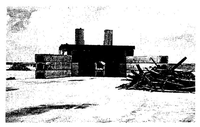
PLATE 22. INCINERATOR FOR WOOD DUNNAGE
