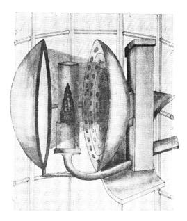
Figure 1. Winslow Lewis' Lamp with Reflector and Lens<sup>15</sup>
