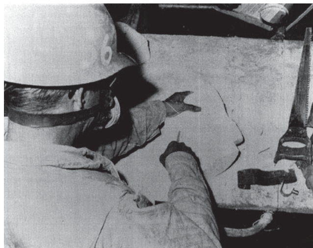
Figure 6. Insulator shaping a piece of insulation at Puget Sound Naval Shipyard. Photo source: Carl Mangold. Previously published in Hollins et al., 2009.
