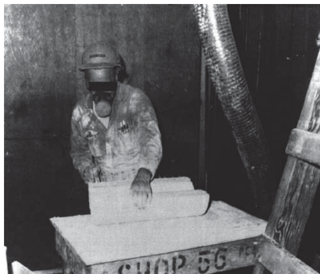
Figure 4. Local exhaust ventilation in the work area of an insulator sawing pipe insulation. Photo source: Carl Mangold. Previously published in Hollins et al., 2009.
