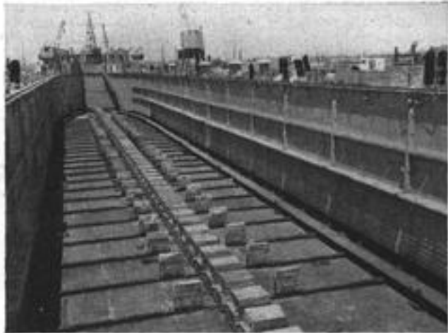
BASIN OF ARD is large enough to accommodate LSTs. This inboard view, looking forward, shows how basin looks empty.
