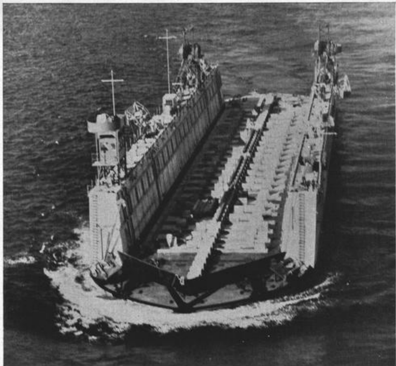
DIFFERENT from ARD on opposite page is this floating drydock, self-propelled and made of concrete. Blocks and underbracing to cradle ships it will service are already installed. Below are other floating drydock types in use.
