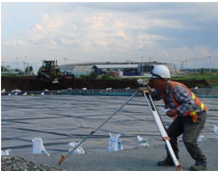
Surveying the limits of excavation in Sen Lake (Photo: TetraTech)
