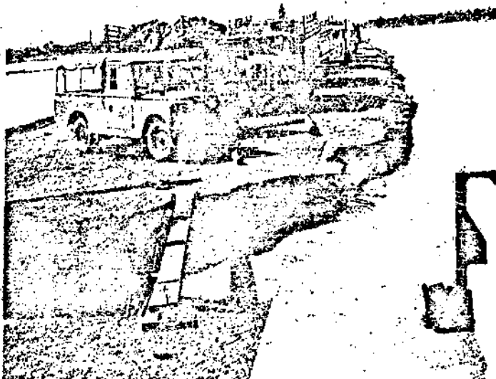
FIGURE 12. COMPLETED WOODEN BARRIER IN PLACE AND BACKED-UP TRUCKS AT WASHOUT
