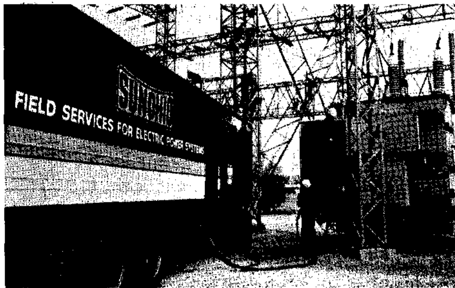
Mobile Sunohio unit cleans PCB-contaminated transformer oil on site
