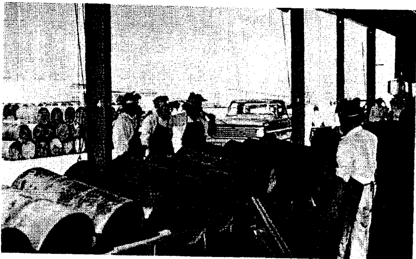
PLATE 13. SAFETY EQUIPMENT. TAKEN IN DEDRUM FACILITY, SHOWING RESPIRATOR, FACE SHIELD, GLOVES AND APRON
