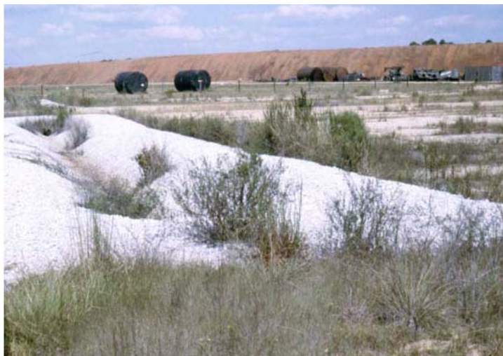
Figure 7.15 A 1980 photograph showing the stabilization of the ditch banks and the re-vegetation of the former Herbicide Orange Storage Site on the NCBC (Photograph courtesy of A.L. Young)
