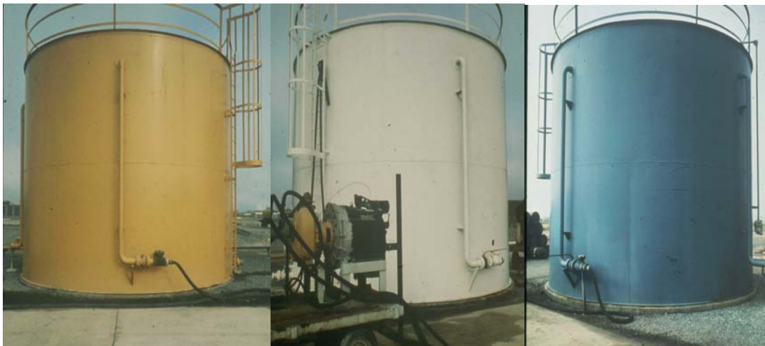
Figure 3.14 Photographs of the 30,000-gallon (113,550-liter) above ground tanks constructed at Bien Hoa Air Base in December 1969 for the temporary storage of Agents Orange, White, and Blue, respectively. Each tank was color-coded to identify the herbicide contained. (Photographs courtesy of J. Ray Frank, Frederick, Maryland)
