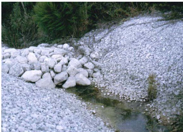
Figure 7.15 A 1980 photograph showing a rock-constructed dam in the draining system leading away from the former Herbicide Orange Storage Site on the NCBC (Photograph courtesy of A.L. Young)
