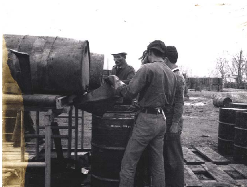
Figure 4.8 Transferring Agent Orange from damaged drums to new drums. South Vietnamese soldiers provided support for the re-drumming operation, Da Nang Air Field, 13 January 1972 (Carmichael Journal 1972)
