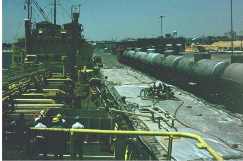
Figure 4.28 During the operation at Naval Construction Battalion Center in June 1977, the Agent Orange was transferred to rail cars and moved to the Port at Gulfport, Mississippi where it was loaded onboard the Incinerator Ship, M/T Vulcanus (Photograph courtesy of USAF OEHL, Brooks AFB, Texas)
