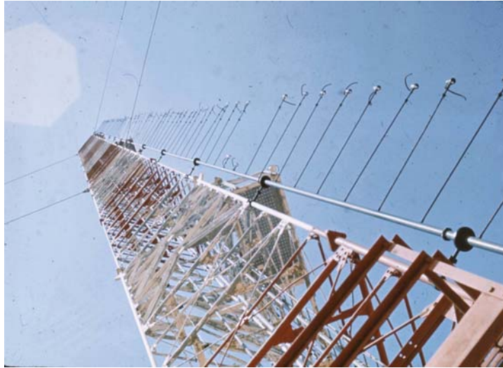
Figure 6.5 The 90-meter tower in the center of Test Area C-52A used for collecting dispersion and wind data in support of Spray Equipment Test and Evaluation Missions, Eglin AFB, Florida, 1969 (Photograph courtesy of A.L. Young)
