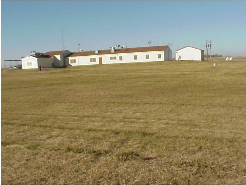
Figure A-0-3. View of Former Missile Alert Facility A-0, Looking East
