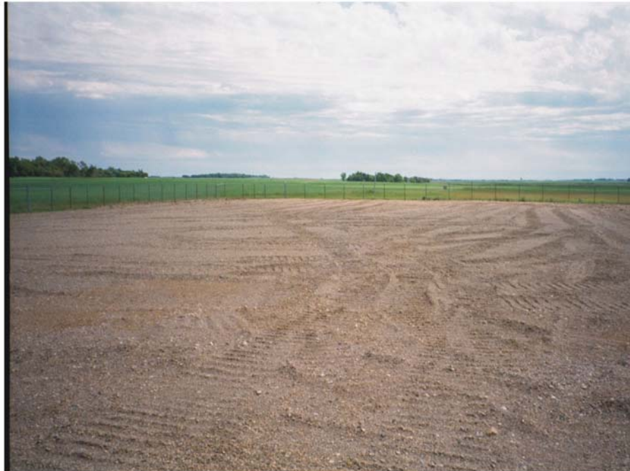
View of Typical LF After Surface Grading, Showing K-04
