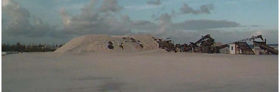
Figure 9 "Above" Pile and SGS Equipment
