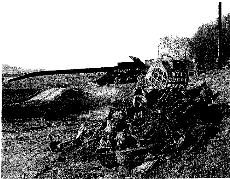
Construction and metal debris
