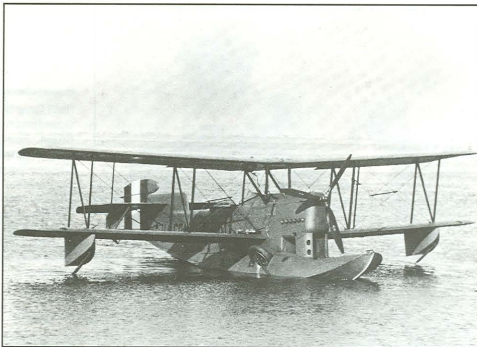
The first aircraft built for the Coast Guard was this Loening OL-5, delivered in 1926. Aircraft were useful in many facets of Coast Guard work, not the least being the spotting of rum boats at sea.
