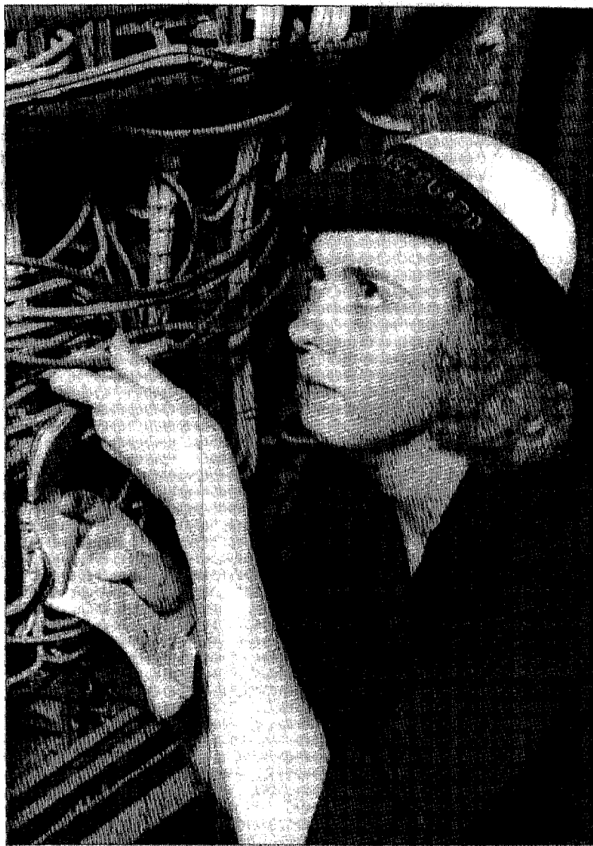
Left: An electrician's mate traces an electrical distribution path.
