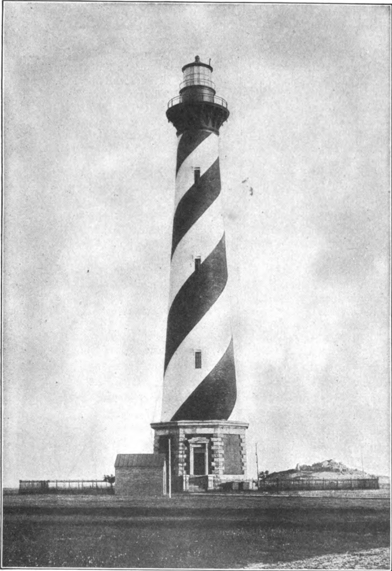
Cape Hatteras Light Station, N. C.
