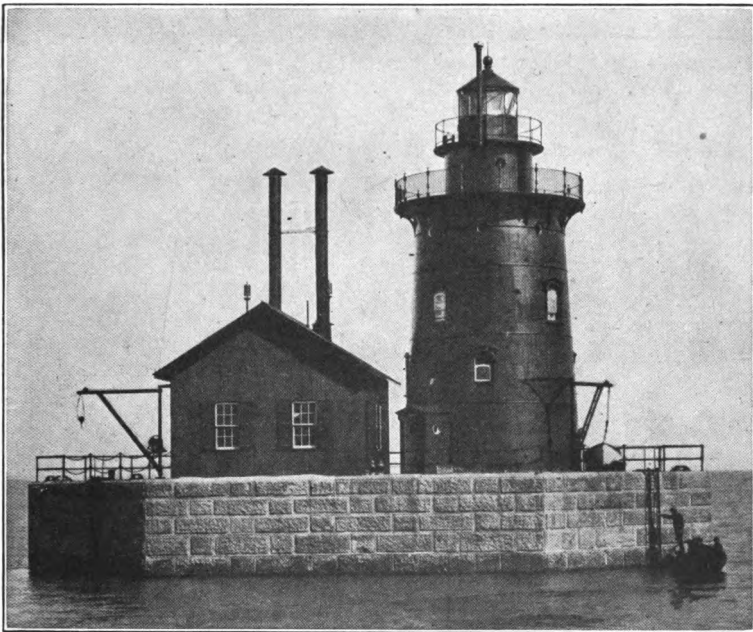
Detroit River Light Station, Mich., showing fog signal.
