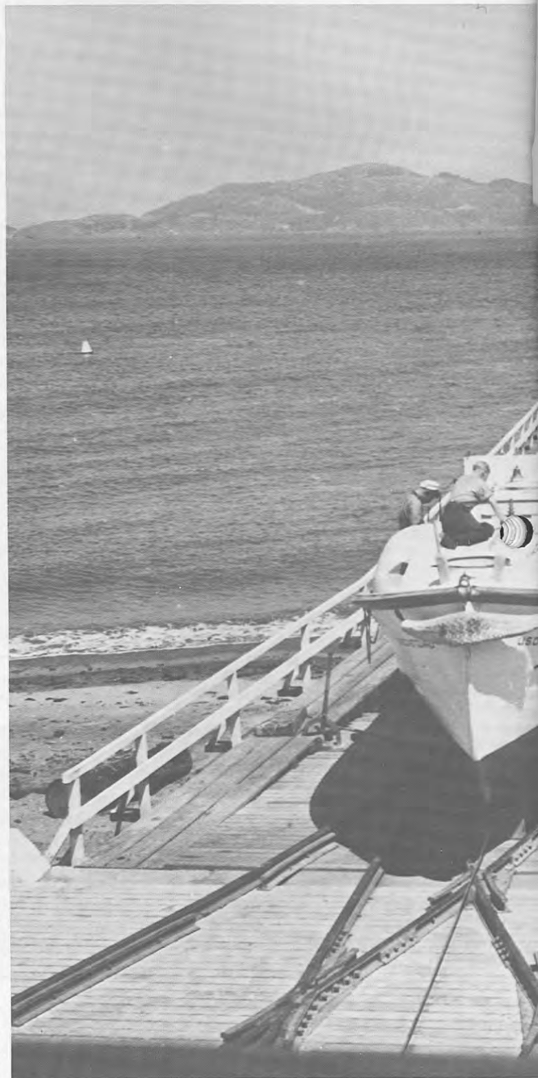
This 1942 photograph clearly illustrates the marine railway at
