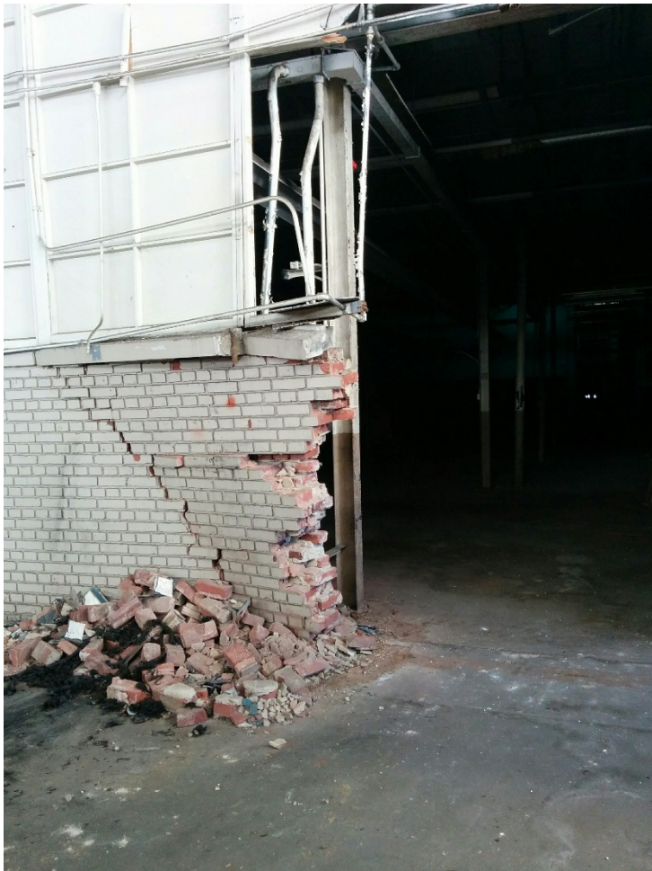
Photo 5 (left). Collapsing interior wall on Building No. 4. Source: DPH, October 25, 2016.
