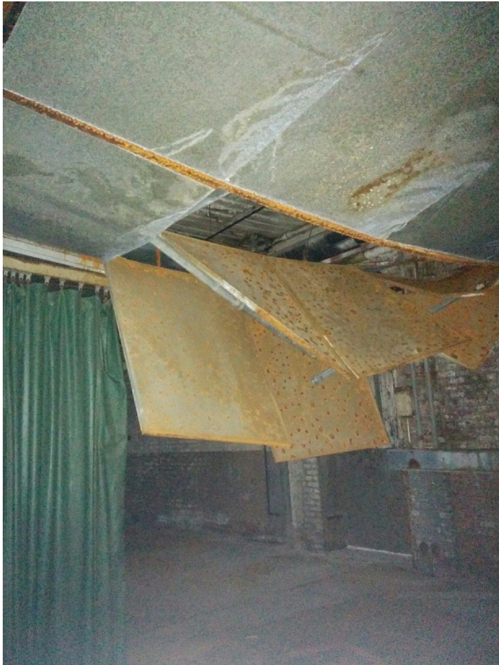
Photo 3 (left). Collapsing roof in Building No. 2. Source: DPH, October 25, 2016.
