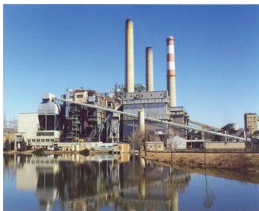
The Xcel Energy Cherokee Station. SOURCE: Photo courtesy of Xcel Energy ( www.XcelEnergy.com )
